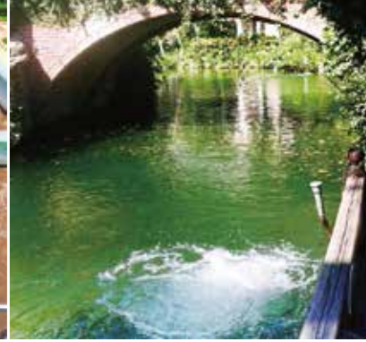
▶ Water circulation and oxygen supply : installed at one meter depth
