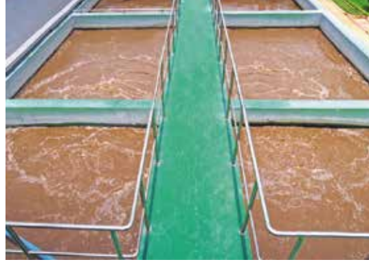
▶ Wastewater treatment: installed at 4.5 meter depth
